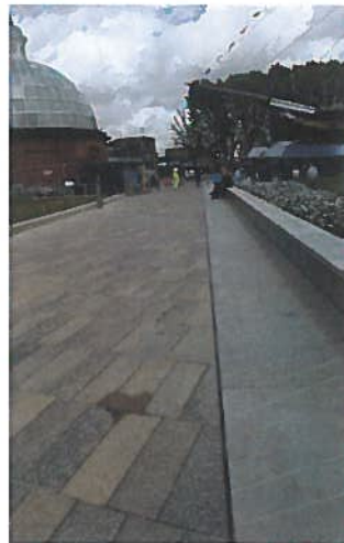
Figure 15 – Slot drain examples: ACO Technologies Plc Slimline and Q-max installation examples. www.aco.co.uk
