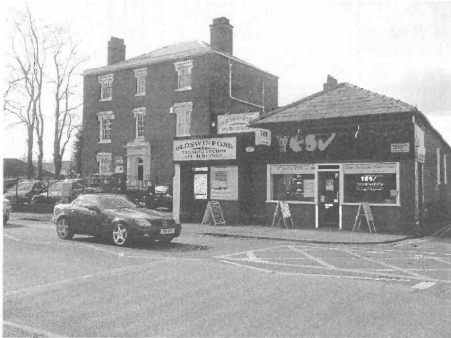
Photograph C. Buildings at the southern end of the centre – shows the attractive character of a number of the buildings
