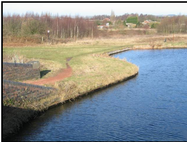
Fishley Junction from the roving bridge – the first five metres or so are retained as a winding hole
