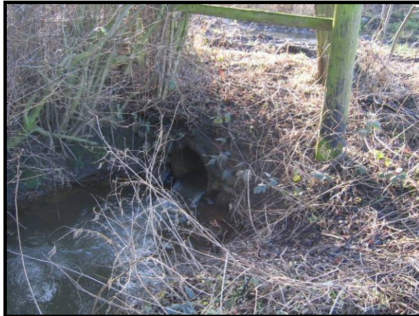
The existing culvert at chainage 9+110
