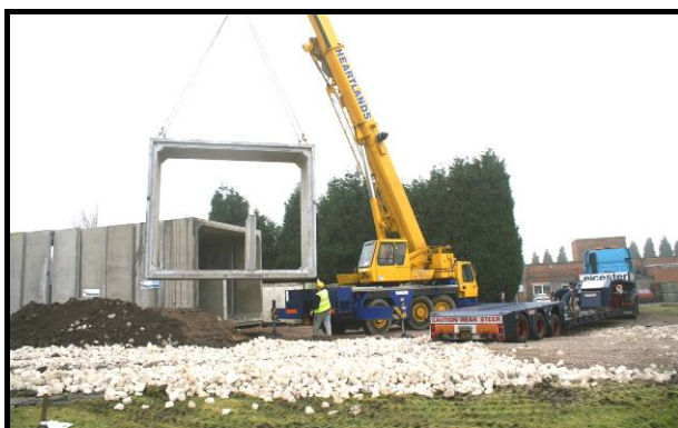
Culvert units already owned by the Trust (purchased with ERDF funding) and suitable for the bridge at chainage 8+410)
