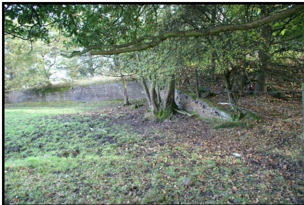
The former tramway retaining wall
