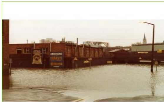
Figure 4-3 Historic flood event 3
