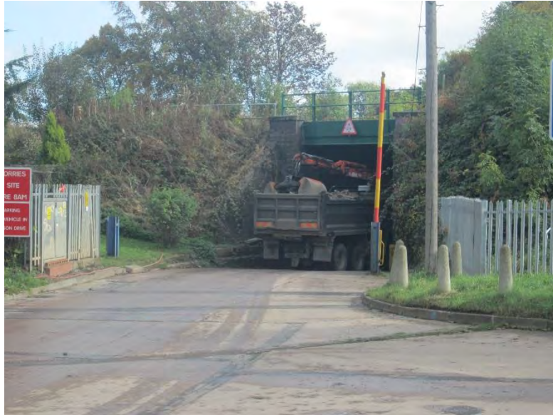
Single lane access under bridge.
